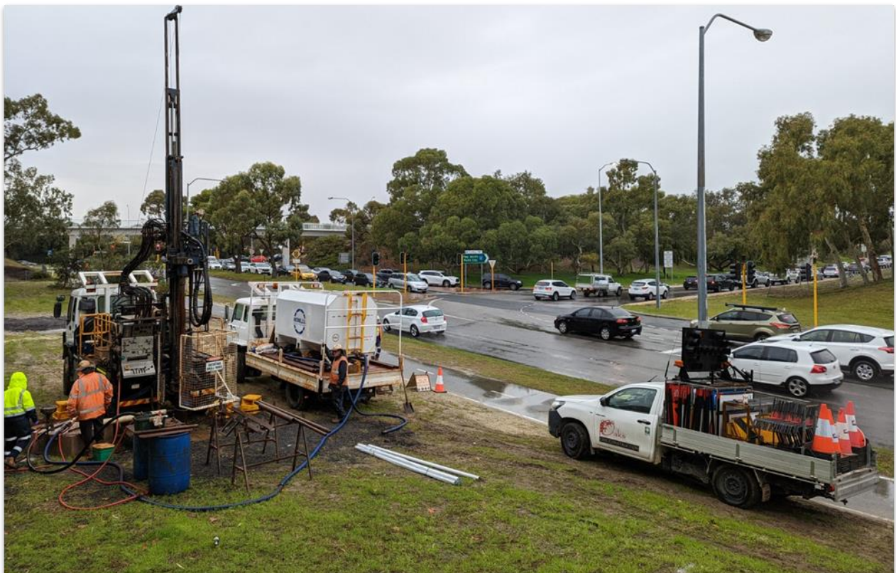
Figure 8 Pre-construction Bore Investigation on Site
